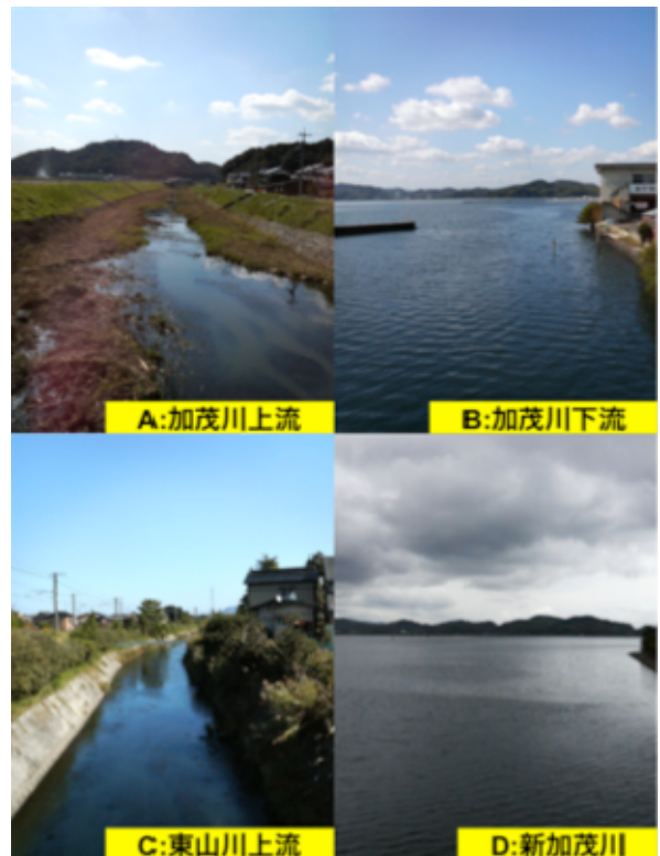
Figure 1. Outward appearance of the A-D observation points.
